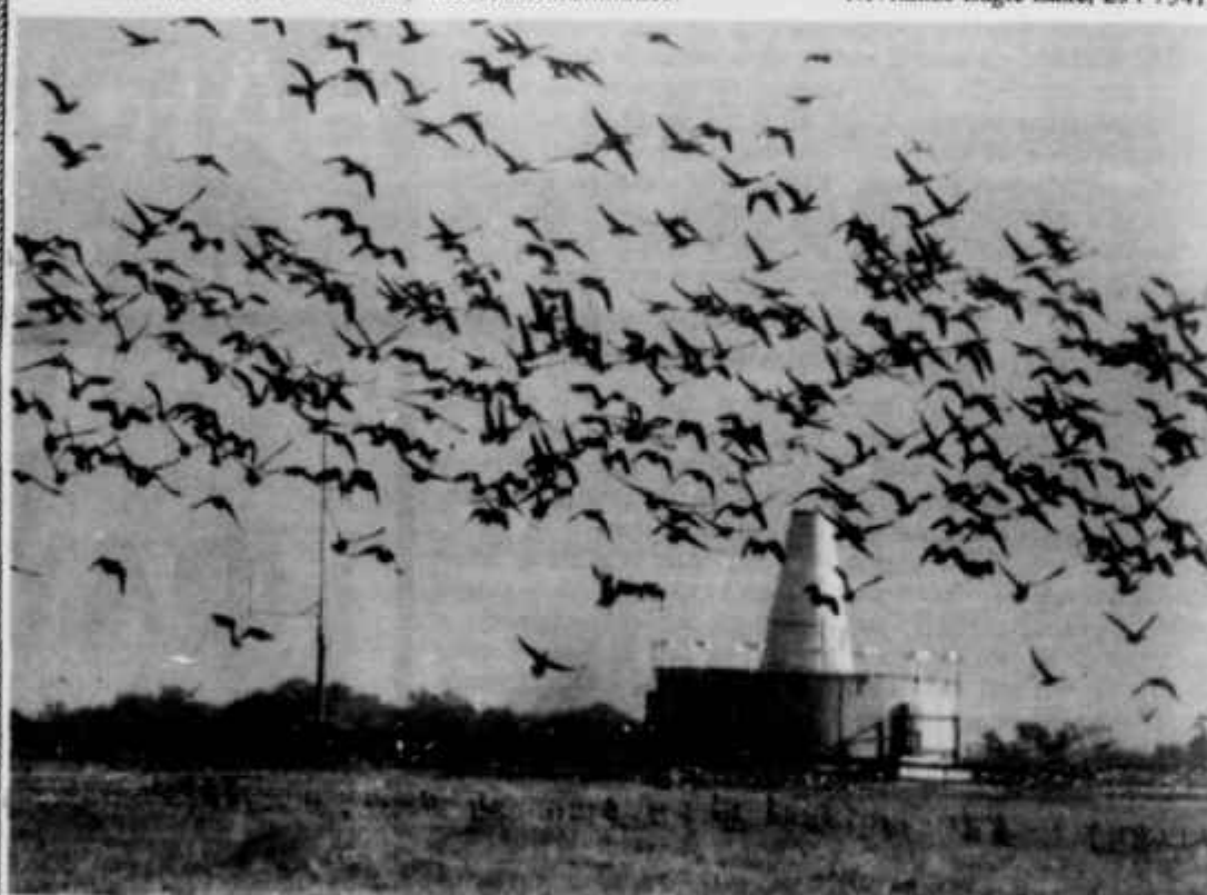
This Omni Station, located at Eagle Lake Municipal Airport and maintained by the FAA, is the only one between Houston and San Antonio.
